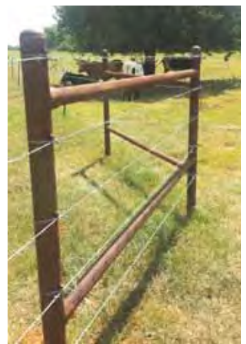
Pre-saddled pipe sleeves save time and make welding pipe fence easier.
