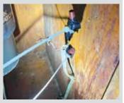
"I capped live wires and wrapped both ends of the tape on the wire itself. Then, I put a cable tie over the ends. Hopefully, this will hold the tape after it ages and the glue goes bad."
