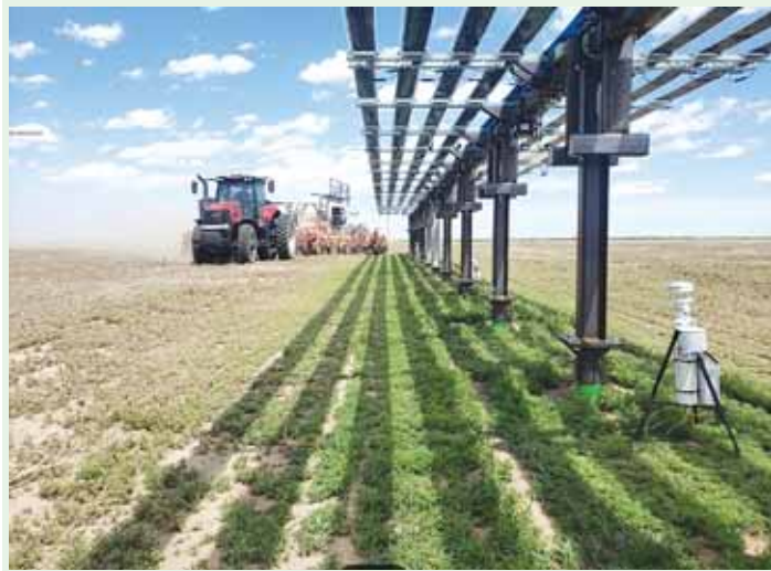
Through the course of the day, the entire rack rotates to a horizontal plane at midday and faces west in a near-vertical plane at sunset.
