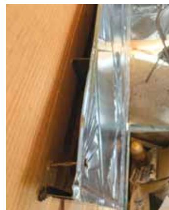
Metal is spaced 4 in. from wood walls and with a 5-in. bottom gap to circulate heat away from walls.
