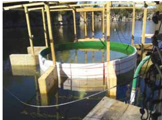
Nearly finished floating fish tank with outriggers.
