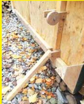
I made this gate stop for the wooden shed where I keep my firewood. It consists of a wooden "stop" that pivots down to the ground to hold the gate in place. When not in use, it pivots up and is held in place by a bolt attached to a round wood handle. **(Richard Mountcastle, Rockville, Ind.)**
