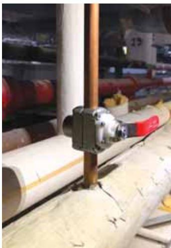
With the EasyFit valve, you don't need to shut off water or freeze lines to make repairs.
