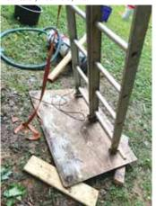
"We took a rigid piece of 3/4-in. plywood and blocked it level with pieces of wood and then screwed the blocks to the plywood with drywall screws. Then we placed an anti-skid strip on top and tied the two ladders together at the top. We added a ratchet strap at 6 ft. The men were up there most of the day and said they appreciated having a solid platform to work from."
