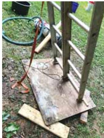
"We took a rigid piece of 3/4-in. plywood and blocked it level with pieces of wood and then screwed the blocks to the plywood with drywall screws. Then we placed an anti-skid strip on top and tied the two ladders together at the top. We added a ratchet strap at 6 ft. The men were up there most of the day and said they appreciated having a solid platform to work from."
