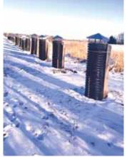
The field end of each pipe begins 3-ft. above ground and is rain capped to keep out birds and debris while allowing air to flow into the underground pipes.
