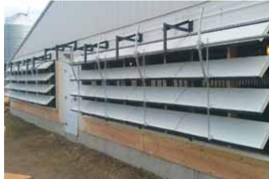
Their unique rack and pinion drives are fitted with limit switches providing the exact torque and speed to properly operate the shutters.
