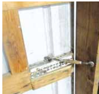
Locking system uses a turnbuckle to adjust door position.
