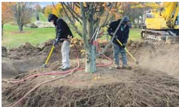
AirSpades are used to blow dirt from roots of tree making transport lighter and easier.
