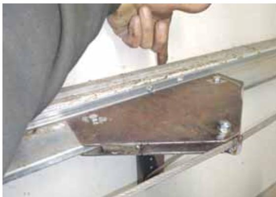
McLaen fabricated a bracket out of two steel plates sufficiently spaced to sandwich the door's top wind reinforcement channel.
