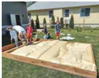
Foley's building is built like a regular shed except for the buoyant foam which they pumped into the spaces between the floor joists.
