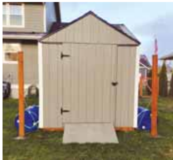
They also added metal posts and chains at each corner of the exterior to keep the shed from floating off to the neighbors.
