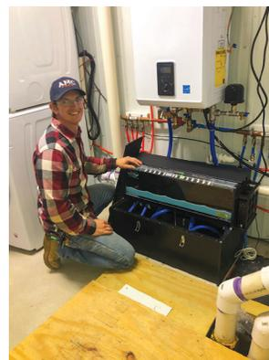
**HUG Hydronics system can be adapted to different sizes and utilize multiple thermostats and zones.**
