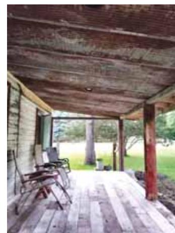
Lance Seltun and Colette Finne used wood beams, planks, and corrugated sheathing from an old barn to make a comfortable overhanging porch on their house.
