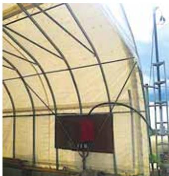
Spare tubing, an old TV antenna and other miscellaneous parts were welded into an electrical pole for a hoop building.
