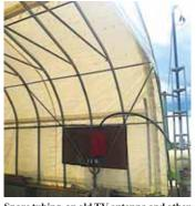
Spare tubing, an old TV antenna and other miscellaneous parts were melded into an electrical pole for a hoop building.
