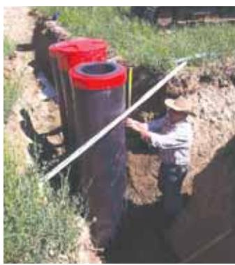
**The columns measure 8 ft. in length and are buried in the ground to a depth of just under 7 ft. leaving approximately 20 in. sticking up out of the ground.**
