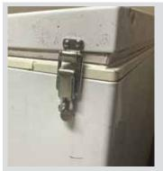
Kylidge McNally, Bethune Saskatchewan: "The seal was worn out on the deep freeze in our house, causing the lid not to seal properly and the inside to frost up. I put a pair of toolbox latches on the lid, one on each side, now it seals up tight."
