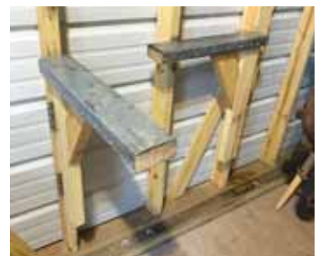
Hinged brackets made from treated lumber fold flat against wall when not in use.
