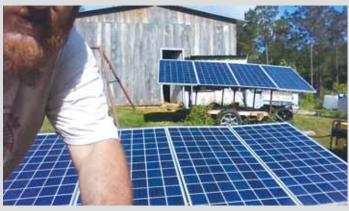
The ground-mounted systems for Mull's home and shop are capable of producing  $33,\!000~\rm kW$  a day, and can run a 200-amp MIG welder.
