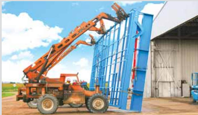
Stand-Alone Door comes pre-assembled in its own pre-squared subframe. Just frame in the opening and slide the door in.
