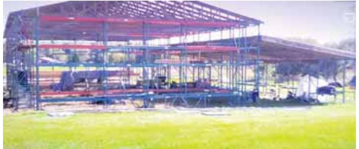
Karkau got 350 8-ft. and 12-ft. pallet rack cross members from an old warehouse for \$400. As a bonus, the price included 100 sheets of 3/4 and 1/2-in. plywood, which he used for divider walls and adding a second floor to his building.
