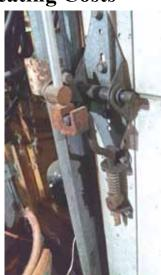
By closing the door, a spring-loaded hook latches into a slot. As wind moves the door, the latching spring will pivot the latches tighter, holding the door tight to eliminate gaps.
