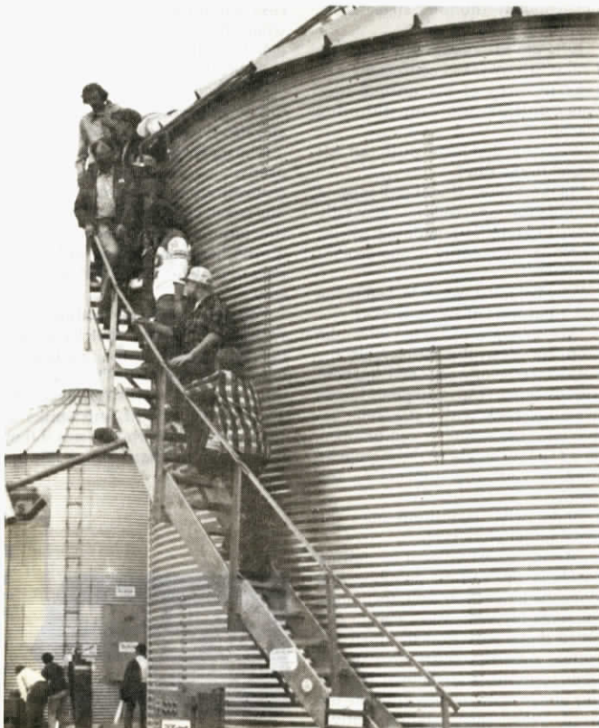
Easy-up stairs can be installed to the right or left. All parts are galvanized.
