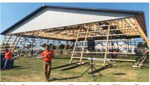
Four 50ton jacks under building raise up roof and sides in minutes.
