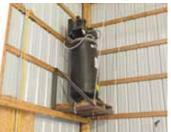
Nitro air compressor is bolted to the wood pallet it was shipped on, and chained to a metal frame that's bolted to corner of building.
