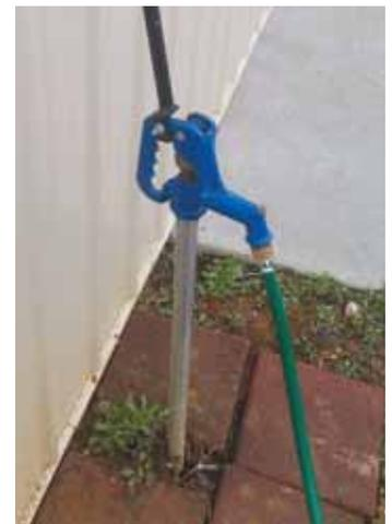
**A 2-ft. long pipe mounted on hydrant handle provides operator with more leverage.**
