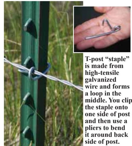
T-post “staple” is made from high-tensile galvanized wire and forms a loop in the middle. You clip the staple onto one side of post and then use a pliers to bend it around back side of post.
