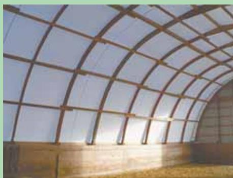
Silver Stream makes hoop barns with either steel or wood hoops. The advantage of wood is that it's easier to insulate and it can be tinned over at any time, if desired.
