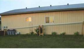
Rainwater drops off garage roof into "half-pipes" mounted on X-shaped wooden supports, and flows into a 300-gal. Rubbermaid tank.
