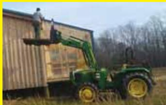
Our loader-mounted, 4 by 6-ft. scaffold comes in handy when constructing new buildings on our farms. Works great for installing siding, windows, vent fans and so forth.
