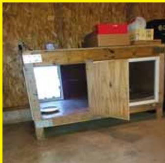
I used mostly scrap material to build a cozy 3-ft. high, 6 by 4-ft. dog house in our garage. It keeps our dog warm in cold weather. The garage wall forms one side of the dog house, and a commercial "doggie door", consisting of 2 clear plastic flaps, leads outside the wall to a step and a plywood windbreak. The doggie door came with an extra panel that can be slid on outside the door to lock it up.
