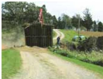
Old bridge deck was removed with a big backhoe and placed temporarily upstream to carry light traffic during construction.
