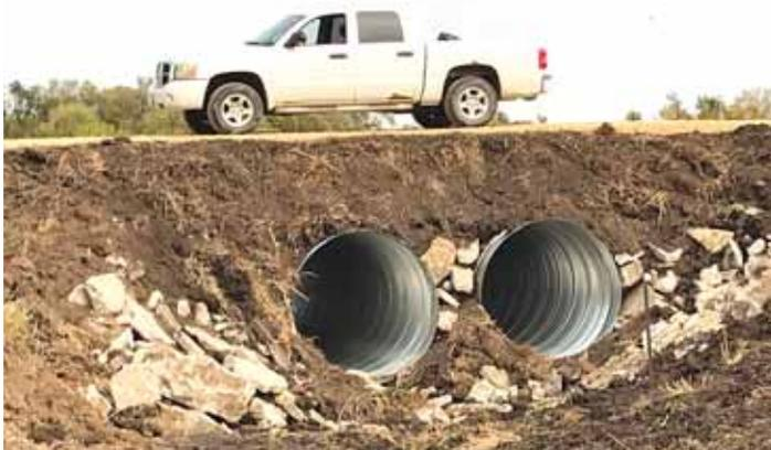
A contractor replaced the 70-year-old bridge on Gogerty's farm road with two 28-ft. long corrugated metal drainage pipes.
