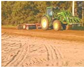
**Farm equipment is all that is needed to prepare the soil and mix the solution. An industrial roller or packer will do the best job compacting. Discs and rototillers may also be used to mix the soil. After the correct grade is achieved, compacting is key.**
