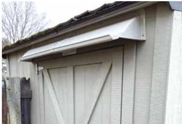
**Rain diverters extend 7 1/2 in. away from wall and come with a front gutter that diverts rain water off to the side.**
