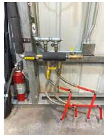
**Wood stove heats an overhead water tank that serves as a heat exchanger. Hot water is then pumped through Pex tubing installed in shop's floor.**
