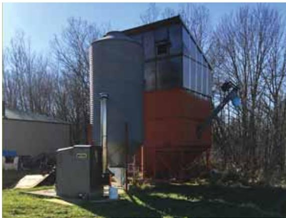
Outdoor biomass boiler can burn almost anything that will feed through a typical farm auger, including old moldy grain.
