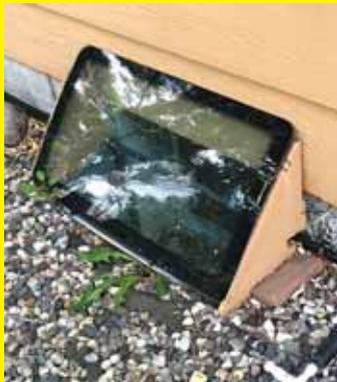
Here's a photo of a window well covering for our house that I made using the tinted glass side window off an old van. The window measures about 30 in. long and 20 in. high, and is just a little wider than the window well. I placed the window against the house at a 45-degree angle, setting the bottom up against the metal window well. A couple of plywood pieces were used to close up both sides.
