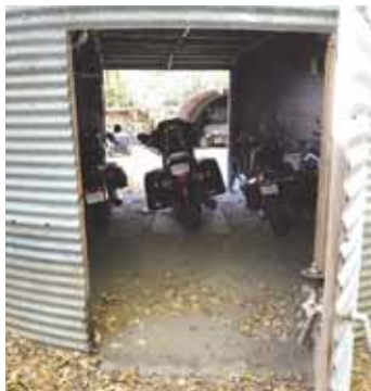
The Ziegler's drive-through grain bin is equipped with a garage door on one side and a cut-out door on the other side.
