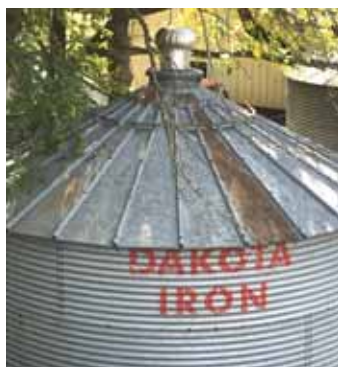
Bin rings were bolted together to build a 15 by 24-ft. portable hoop shed that rides on barn pole skids (above). Roof ventilators installed on firewood storage bins to help dry the wood.
