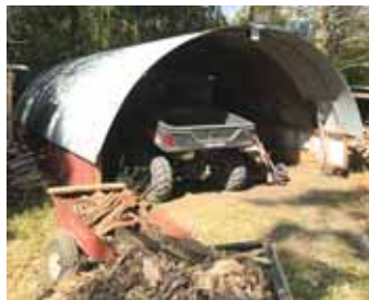
Bin rings were bolted together to build a 15 by 24-ft. portable hoop shed that rides on barn pole skids (above). Roof ventilators installed on firewood storage bins to help dry the wood.
