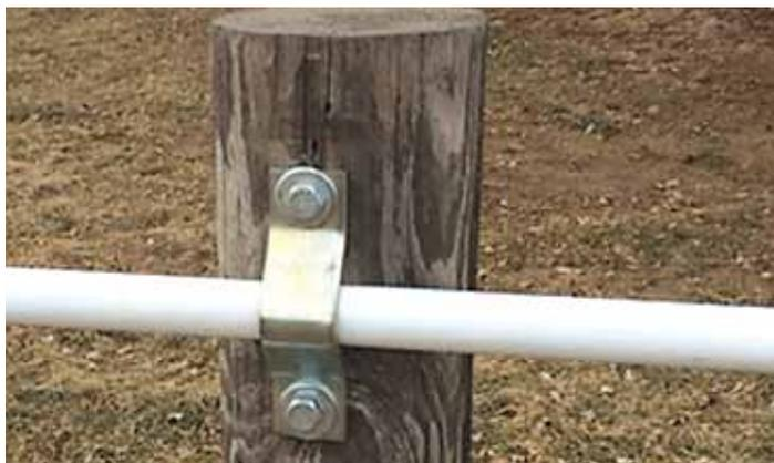
TJ's Fencing surface-mills recycled fiberglass fence tubing and then adds a special coating that prevents slivers.
