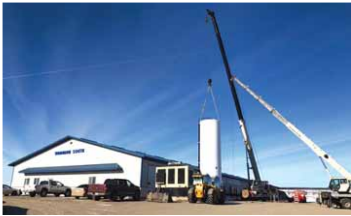
Big 20,000-gal. vertical tank provides 36 hrs. of milk storage, at about two thirds the cost of barrel-shaped tanks.
