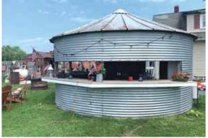
a loader tractor with forks to set the bin on a trailer and haul it home. Their son used a torch to cut the bolts off most of the middle section of the bin, and then removed all the panels for the bar.
