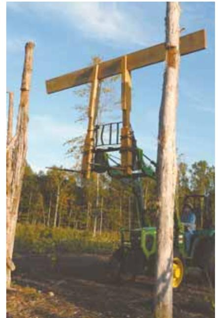
**Agnew uses home-built loader-mounted truss lifter to raise wood beams up to 20 ft. high, then bolts them into notches cut into building's posts.**
