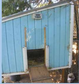
Wooden tracks guide transparent plexiglass door up and down, allowing Hollenstein to see inside when door is closed.
