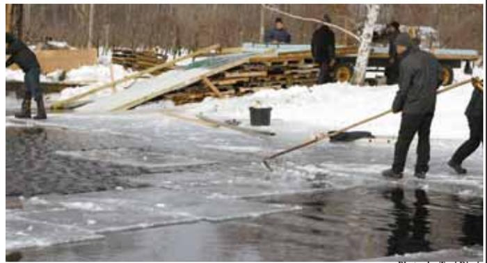
Ice is sliced into 4 by 7-ft. sheets that are 8 to 12 in. thick.
