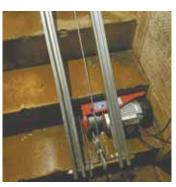
Electric hoist fits under tracks on bottom basement step.
