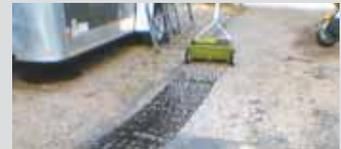
"I use an old drop-down lawn fertilizer spreader to apply asphalt sealer on my driveway. I cover all the holes in the spreader with duct tape, except for the metering holes at the bottom. I fill the spreader about 2/3
