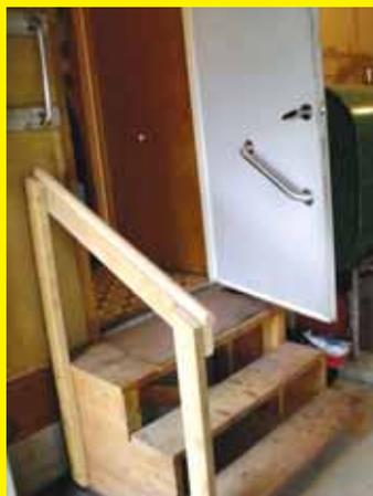
I made another handrail alongside movable steps that lead from the garage to our home's mud room. It's made from 2 by 4's with a round handrail screwed on top of it. I attached a 19-in. long metal handle to the inside of a steel door to provide assistance as my wife walks up the steps. I drilled starter holes, then used large hex screws to attach the handle's flanges to the door. **(John Lubinski, Plainview, Minn. J.J.Lubinski@yahoo.com)**
