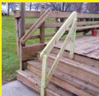
I needed a second handrail on the stairs leading up to our deck so that my wife, a stroke patient, could get up or down the 3 steps. Both sides of the handrail have a 1 1/2-in. wide, 3/8-in. deep recessed finger groove in them. The 2 handrails are about 3 ft. high and 28 in. apart.
