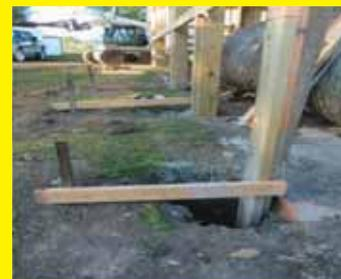
When constructing a building, we attach horizontal 2 by 4's to the 2 by 6 wall studs and to steel posts driven into the ground, to make sure the studs remain upright until the hole gets filled with concrete. By covering the entire base of each post with concrete – instead of just pouring a footing – the posts are protected from rot and anchored securely in the ground. **(Mark Mahlow, 71049 120<sup>th</sup> St., Zearing, Iowa 50278 ph 515 487-7708)**
