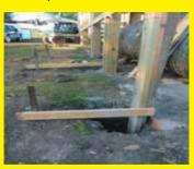
When constructing a building, we attach horizontal 2 by 4's to the 2 by 6 wall studs and to steel posts driven into the ground, to make sure the studs remain upright until the hole gets filled with concrete. By covering the entire base of each post with concrete – instead of just pouring a footing – the posts are protected from rot and anchored securely in the ground. (Mark Mahlow, 71049 120<sup>th</sup> St., Zearing, Iowa 50278 ph 515 487-7708)
